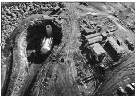
The U.S. Army Corps of Engineers built South Dakota's 15 underground Minuteman missile launch control centers in the early 1960s.
